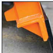
4" x 4" x 3/4" Bottom angle with 1/2" reinforcement gussets every 12"
