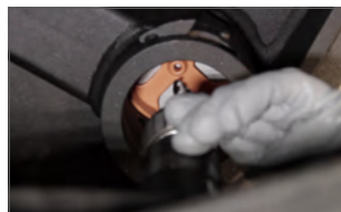
Step 3 - Use Center Locator to drill pilot hole up from under bed
